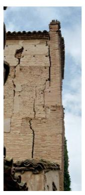
Figure 6: View of major crack in the NE wall
